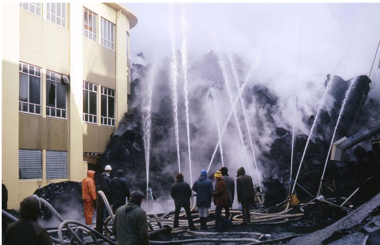
Figure 4: Cold sea water was pumped consistently onto the advancing lava flows. The aim was to cool and solidify the molten material to form a dam, forcing the lavas to find an alternate route away from the harbour. Photo: Sigurjón Einarsson, used with permission.
