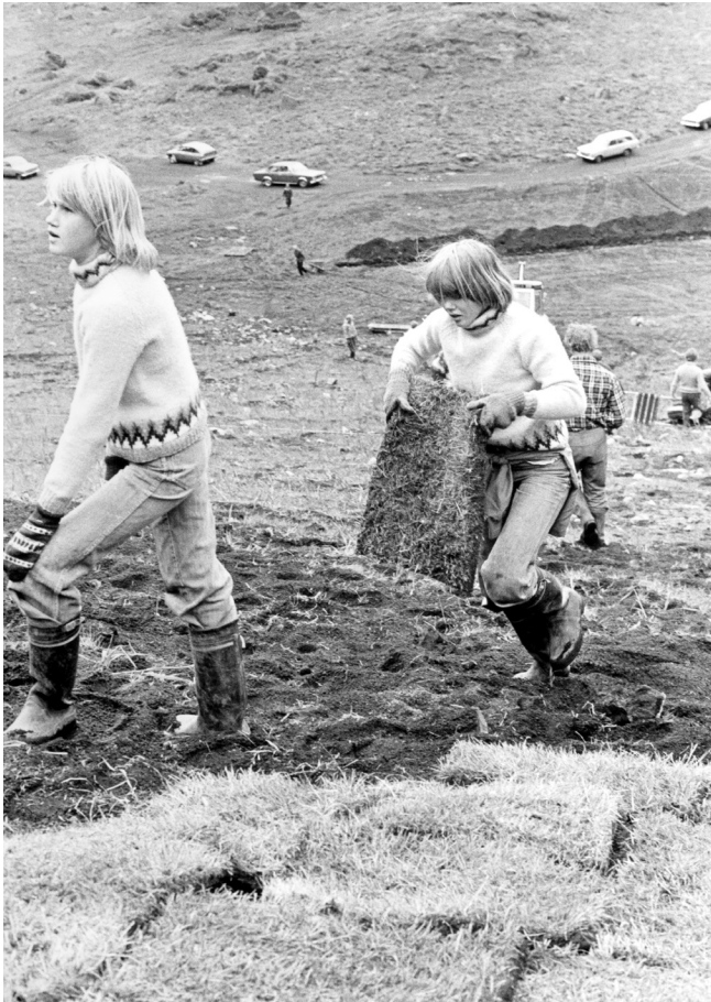
Figure 6: Reclamation work on the island included revegetation of the barren landscape. Revegetation bound the remaining loose ash particles which were being reworked by strong winds, causing further damage to properties and cars. Photo: Sigurgeir Jónasson, used with permission.
