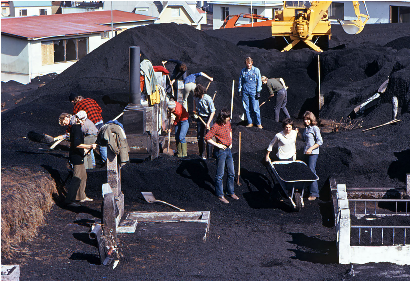
Figure 5: Residents and volunteers cleared 2.8 million m 3 of ash and scoria, which reached depths of up to 3 m, to support the return of the community to the island. Some areas were cleared using machinery and diggers, while other areas such as the cemetery had to be cleared by hand. Photo: Sigurgeir Jónasson, used with permission.
