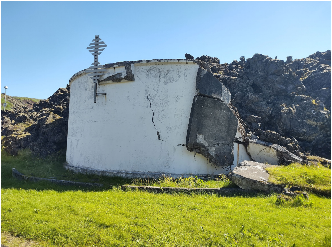
Figure 14: The water tank at Skansinn provided sea water to the local swimming pool and fish factories. The tank was damaged and partially covered by the Eldhraun lavas in 1973. Photograph: Rh. H. Meara.
